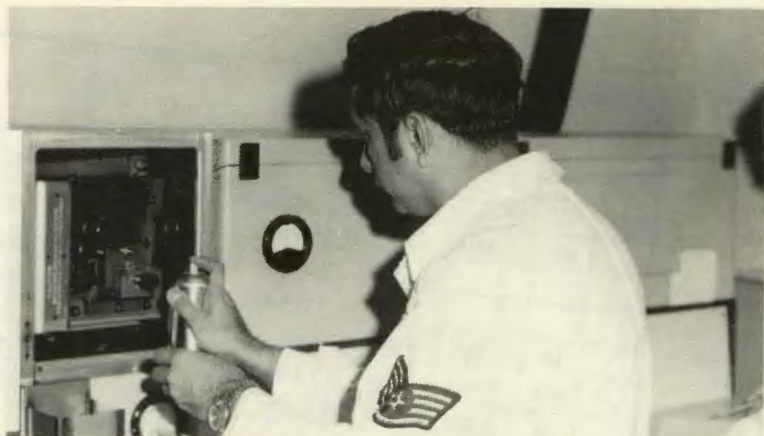
Sample excitation chamber is cleaned prior to next analysis. Chamber and quartz window must be kept clean to insure best possible results.
